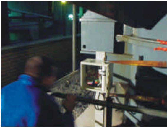
Fig. 3. Hall effect probe (white box) on transformer Earth line (copper) at Hunterston power station. Engineer (lower left) shown for scale.
